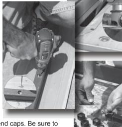
Determine which direction/post you are routing the wire to and tape the wires to the top rail in that direction.
